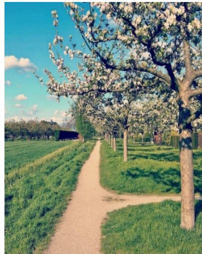
Paden in halfverharding
